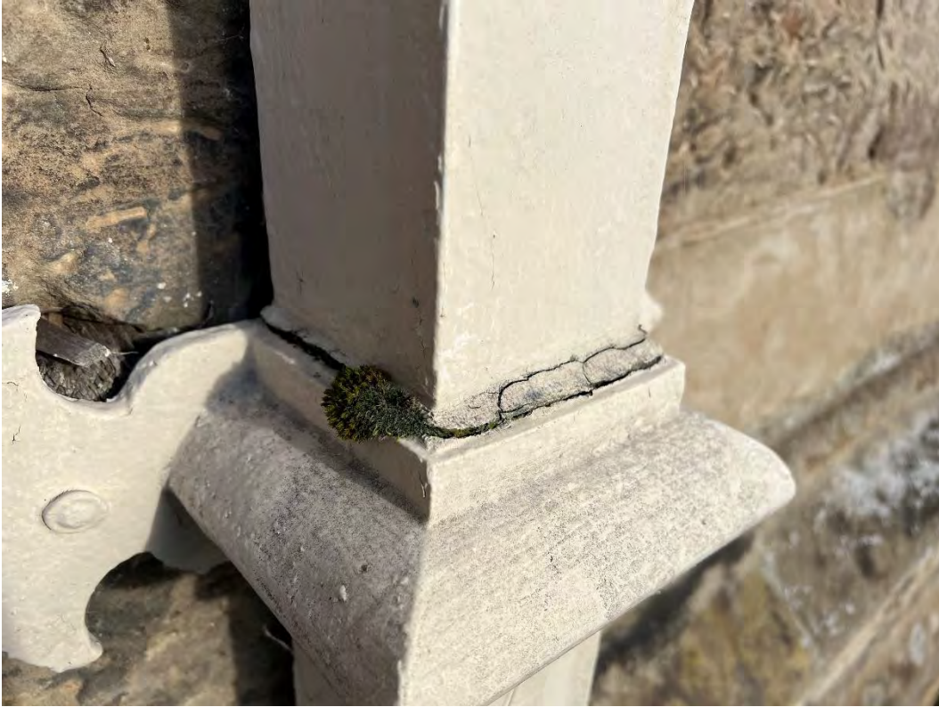
1019) Typical condition of downpipe joints
