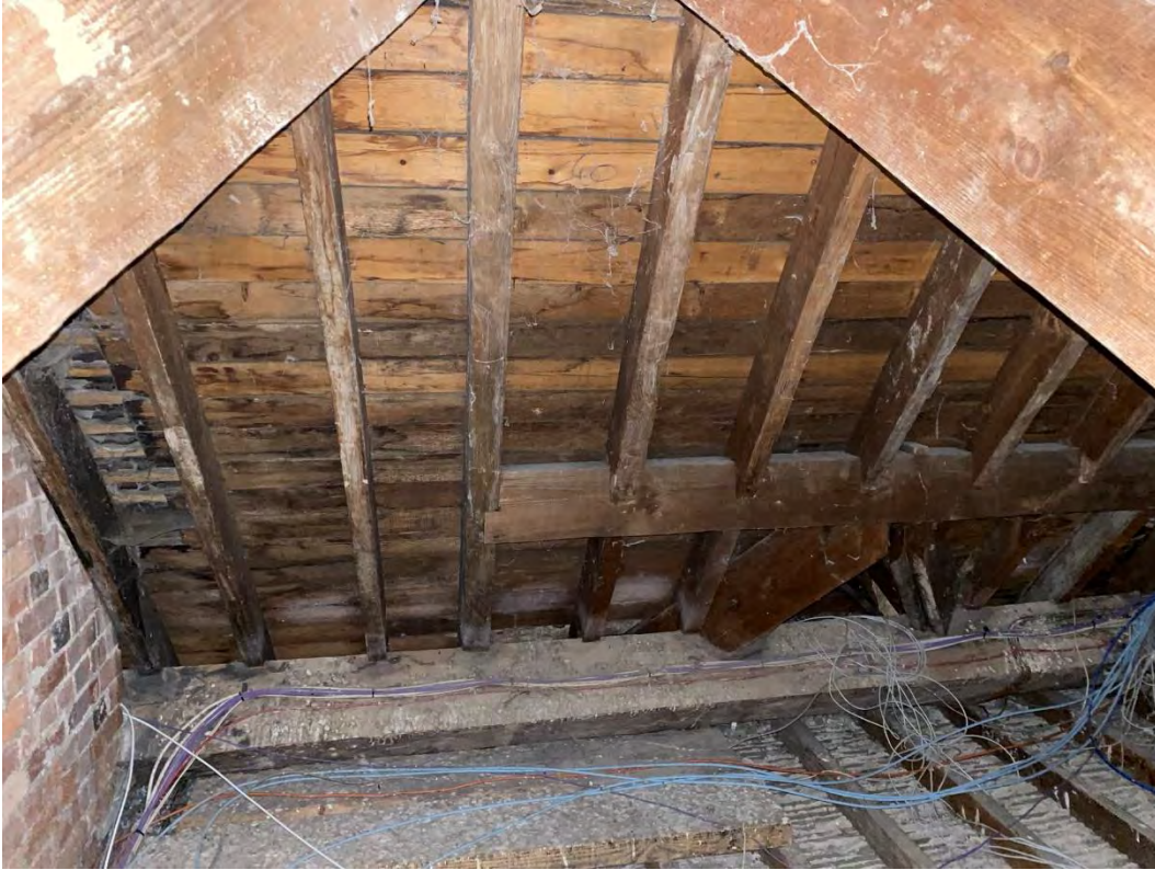
1035) View of internal sarking boards
