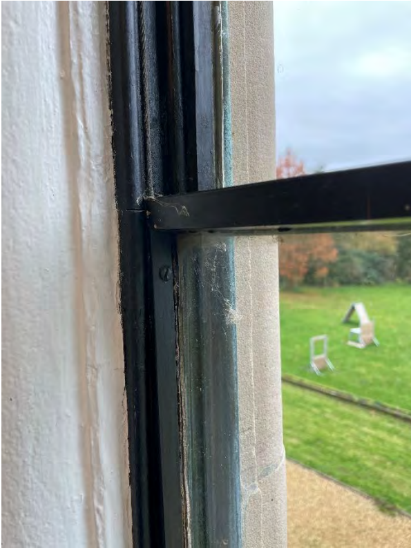
1011) Internal view of typical sash window
