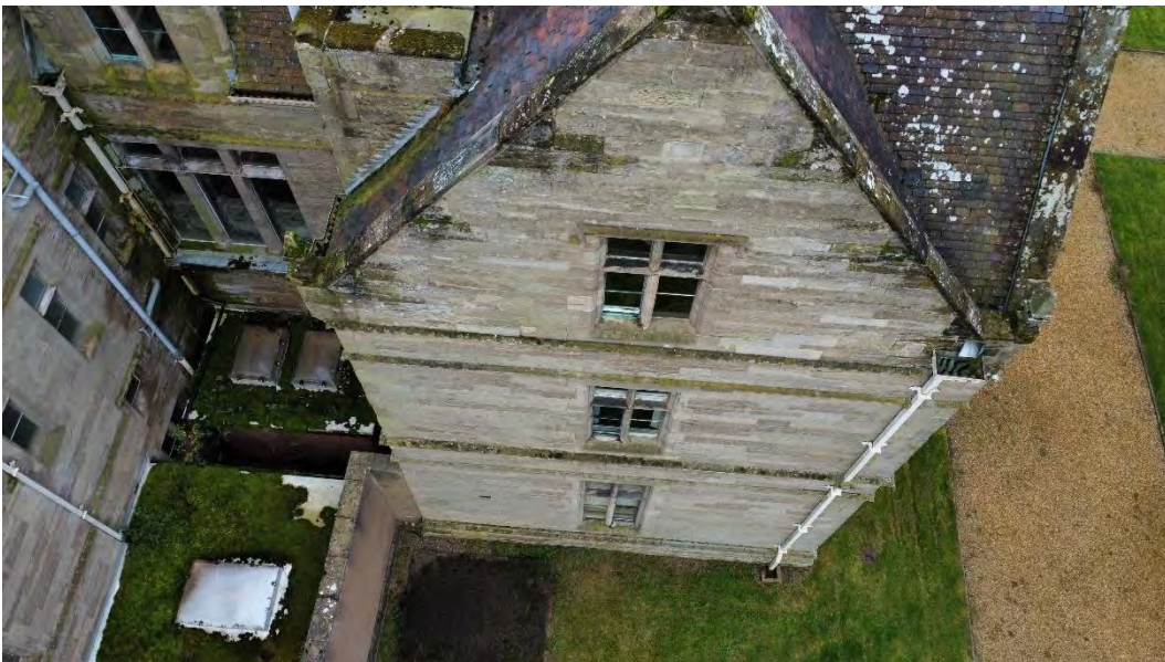
1004) North Elevation (off rear)
