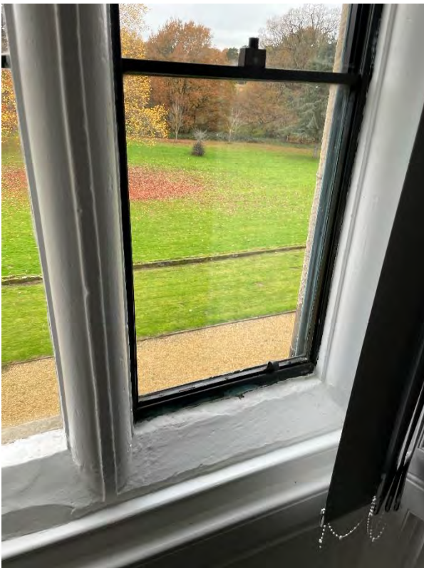
1012) Internal view of typical sash window
