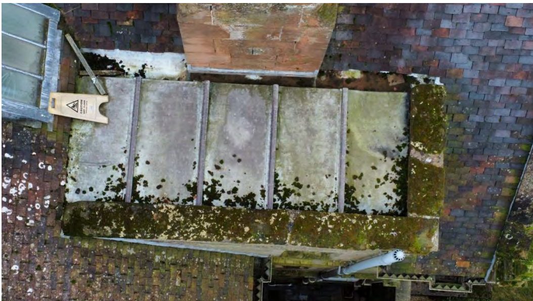
1014) Flat roof to rear pitch of West Elevation RAPLEYS LLP | 7
