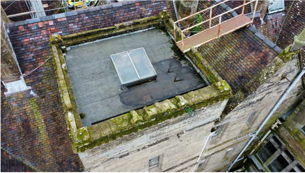
1015) West Elevation - Two Storey Flat Roof
