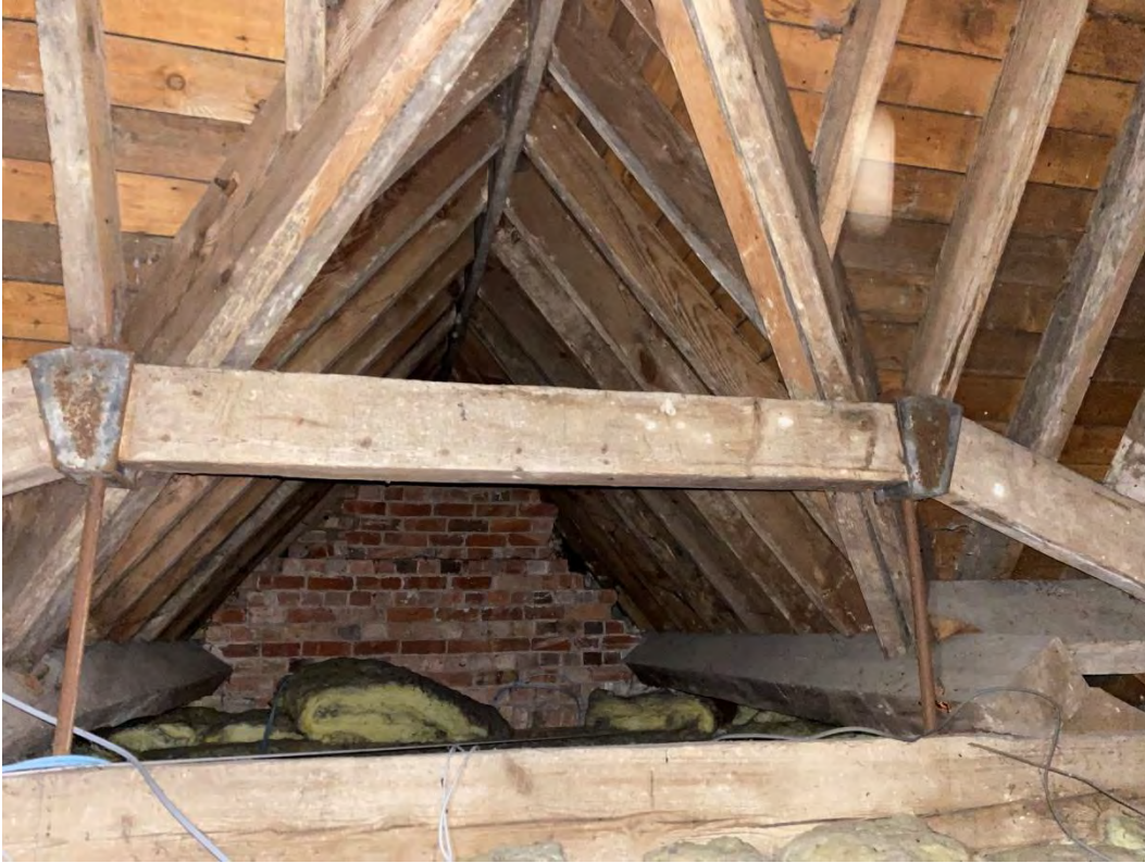
1037) View of retrofitted supports within roof void
