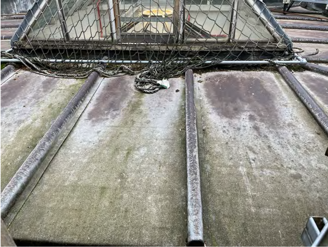
1009) Typical condition of leadwork
